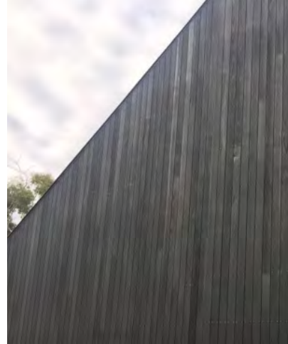
CHARRED TIMBER EXTERNAL CLADDING
